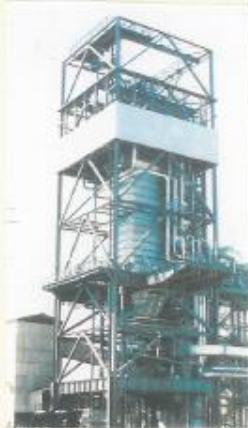
Direct reduction plant
