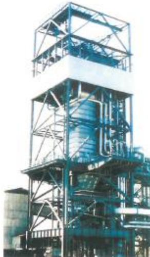
Direct reduction plant
