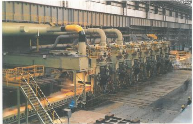
Hot strip mill
